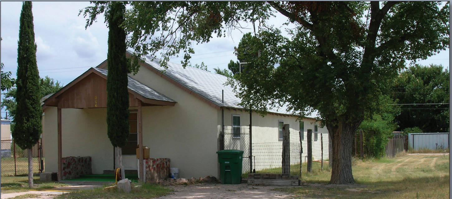
These Two Buildings are Thought to be Former HAAF Barracks that were Moved to Lovington and Converted into Teacher Housing.
