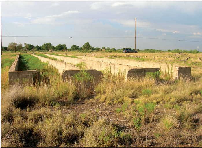
(Clockwise, From the Top) View of the Former Base Hospital Looking North Showing the Concrete Stem Walls that Once Supported a Storehouse, 2007. Rows of Concrete Piers that Once Supported the Hospital Buildings, View to the Northeast, 2007. The Last Remaining Squadron Hangar from the HAAF Era. It was Damaged by a Wind Storm and Demolished in 2005. Looking West along the Flight Line at Vaults that once Housed the Top-secret Norden Bombsights, 2007.
