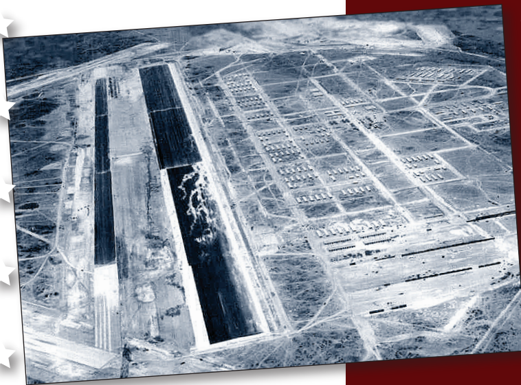
Aerial View of HAAF under Construction. View to the North. Note Completed Barracks to the East of the Runway.
