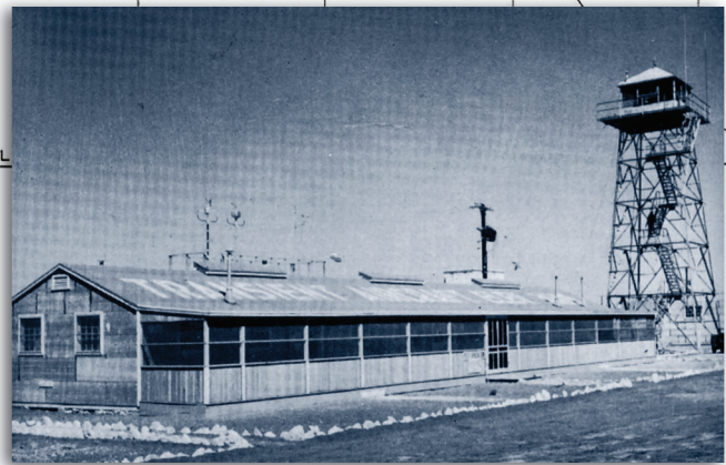
SPECIAL OPERATIONS BUILDING AND CONTROL TOWER
